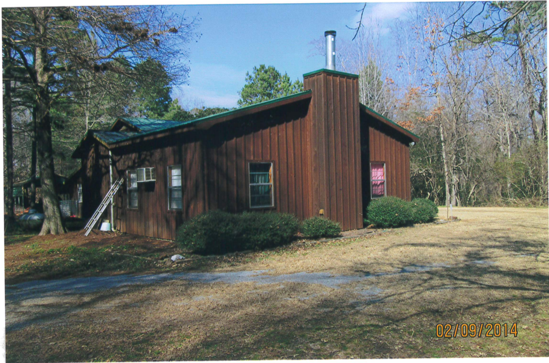
#2, CAMP COOK HUNTING CAMPHOUSE BUILT BY FLOYD COOK 1974
